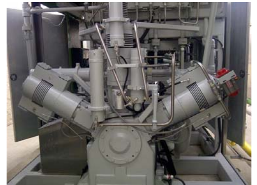
View of Compressor inside enclosure
